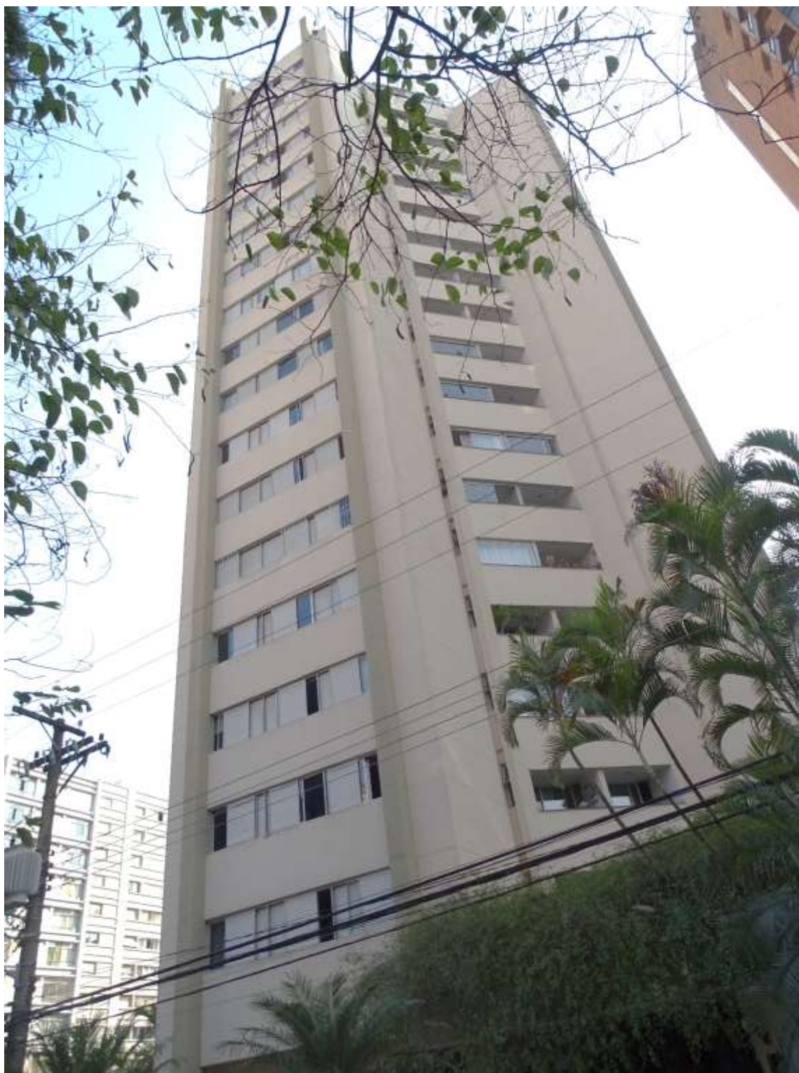
FOTO – 51 – FACHADA PRINCIPAL
